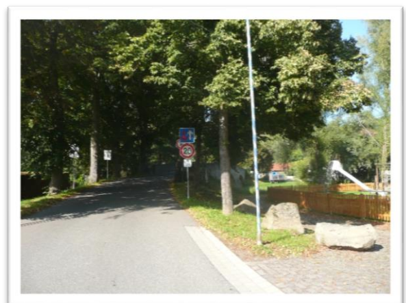
Ahrbrücke in Insul
